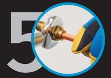
Thread the flare nut onto the male fitting and tighten using correct tools to equipment manufacturer torque specifications.
