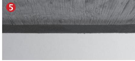
Blaze Foam should be tightly butted together end to end, ensuring there is no open space between two Blaze Foam pieces for all joints and inside and outside corners.
