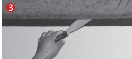
Continue down the length of the joint compressing the Blaze Foam and pushing it into the joint area. To aid in installation, a putty knife or trowel may be used to compress the Blaze Foam and slide it into place.
