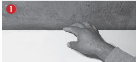
Ensure that the joint area is clean, dry, and clear of any debris or obstruction.
