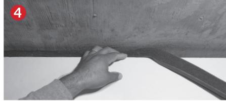
Blaze Foam can be installed flush with the outside plane of the wall or recessed against the top track runner. Ensure the intumescent strip lays flat on the top edge of the gypsum wall.
