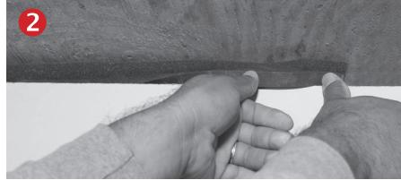
Holding the Blaze Foam with the intumescent strip facing down, compress the foam so that it can be placed within the joint between the top of the gypsum wall and the bottom of the concrete floor above.
